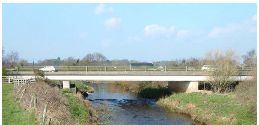
Bridge carrying Castledawson Bypass over the River Moyola
